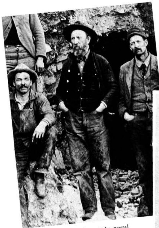
William H. Antrim. Taken at the portal of the Confidence Mine tunnel, near Mogollon, New Mexico, in the 1890s. Courtesy Mr. Elton Cunningham and Corresponding Member H. A. Hoover.
