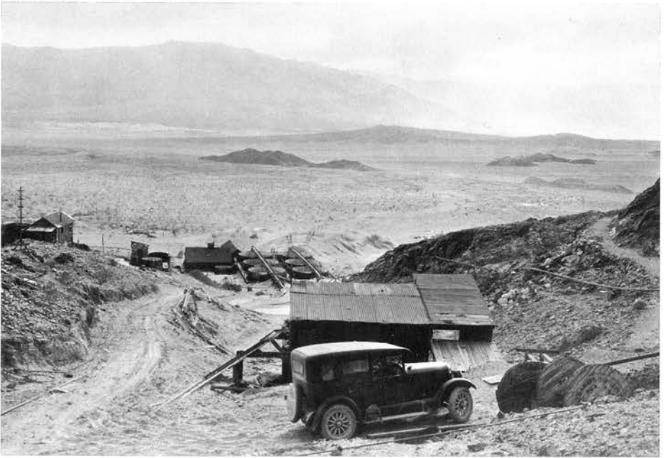
The ruins of the old Keane Wonder Mine in Death Valley with Frasher's photo car in the foreground.
