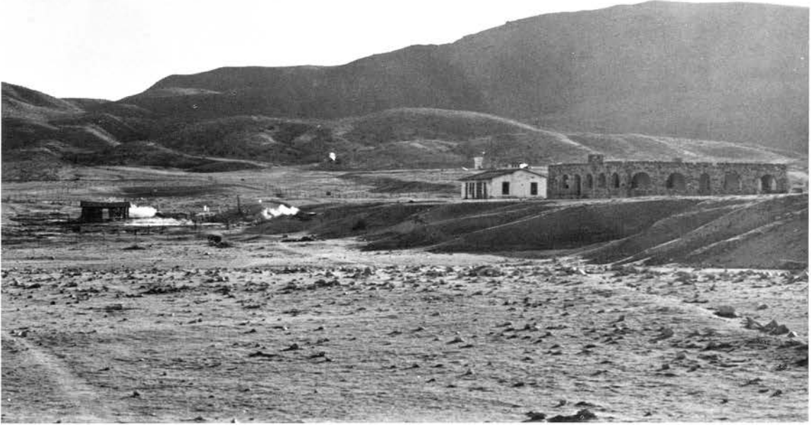
Coso Hot Springs, with its now dormant geysers, abandoned spa buildings and colorful boiling mud pots
