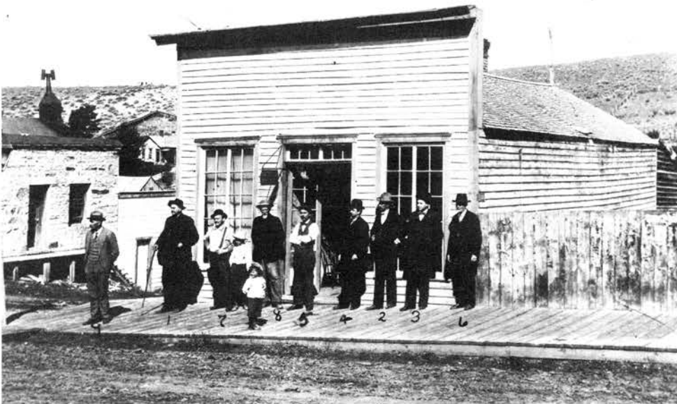
This later drug store was under construction January 14, 1864, and vigilantes used its handy beams to hang five desperadoes, Boone Helm among them.—PHOTO COURTESY MONTANA HISTORICAL SOCIETY
