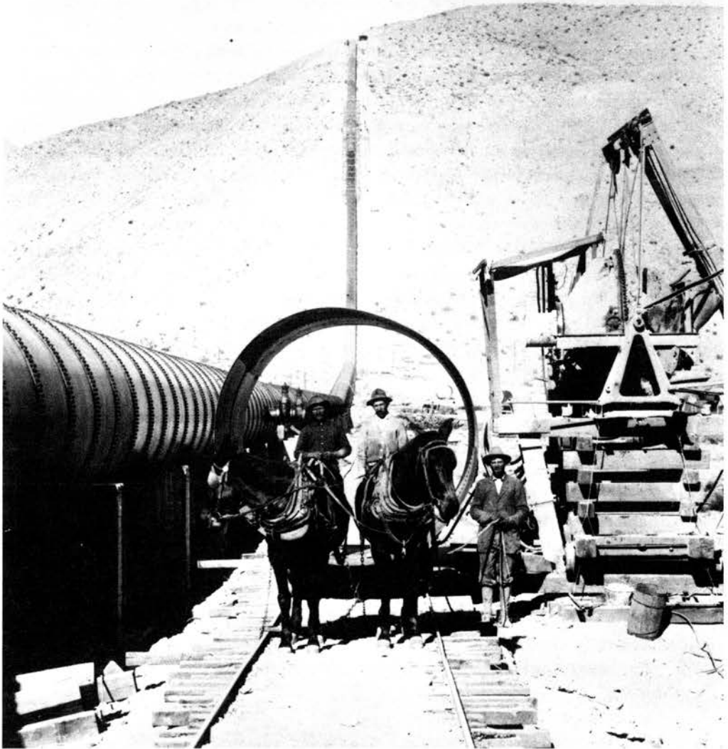
At work on the Los Angeles Aqueduct.
