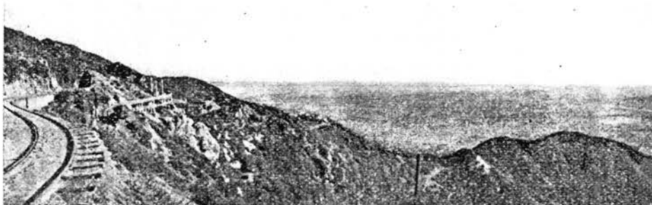
VIEW OF CIRCULAR BRIDGE AND VALLEY. MT. LOWE.
