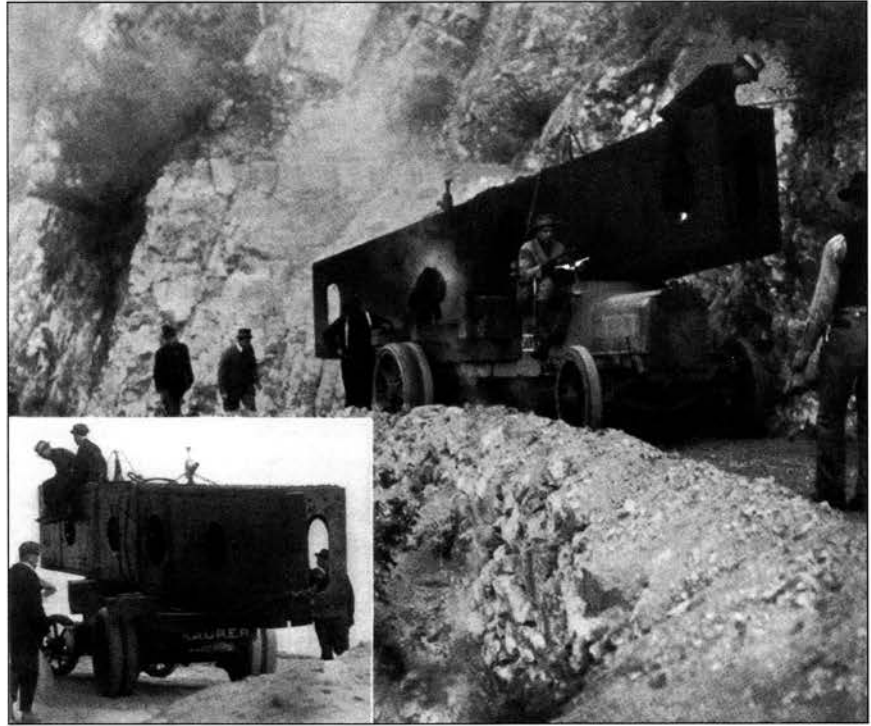
Figure 12. Lower view: backing and filling on a sharp turn. Large view: the rear wheel of saurer crushes through the soft, narrow roadway on the brink.
