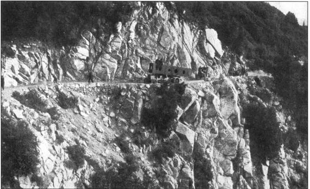
Figure 11. A large boulder weighing twelve hundred pounds fell from the side wall, striking the girder. Note the boulder in the road in front of the second truck.
