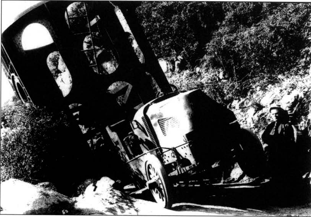
Figure 13. Near-disaster when the road collapsed beneath a Mack Truck hauling part of the tube assembly, for the 100-inch, to the summit.
