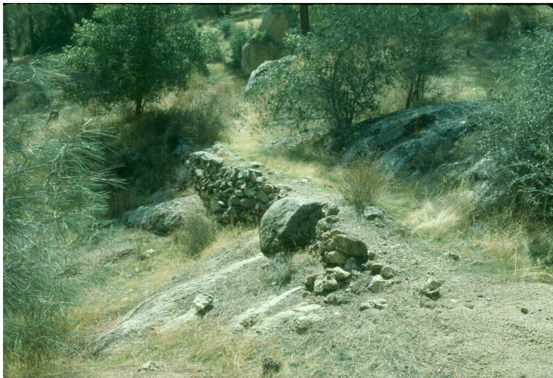
Figure 6: Pack-mule path in the Greenhorn Mountains near Keyesville, dating from the mid-1850s. Note the dry-laid masonry revetment where the path crosses a deep gulch. Such pathways were built and maintained to get crushed gold-bearing quartz from simple arrastras down to lower elevations where enough water was available for gold extraction. After the introduction of stamp mills in the late 1850s, accessed by much more elaborate wagon roads with more gentle gradients, these old mule paths were abandoned. B. Dillon photo, 1983.
