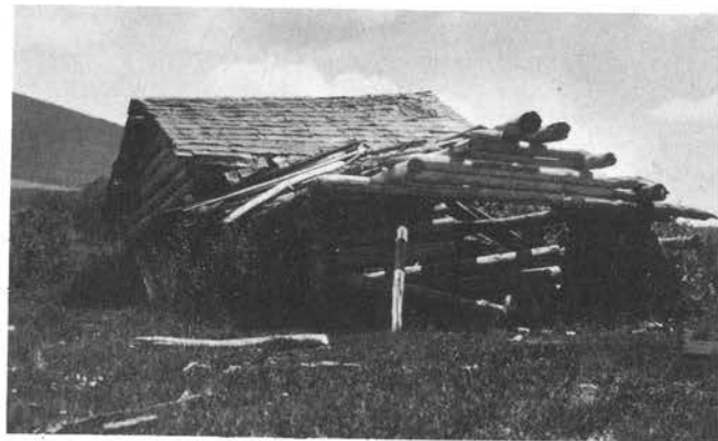
RUINS of the bunk and cook house at the old Bucklar Ranch on the Hart Prairie. Taken in 1926.
